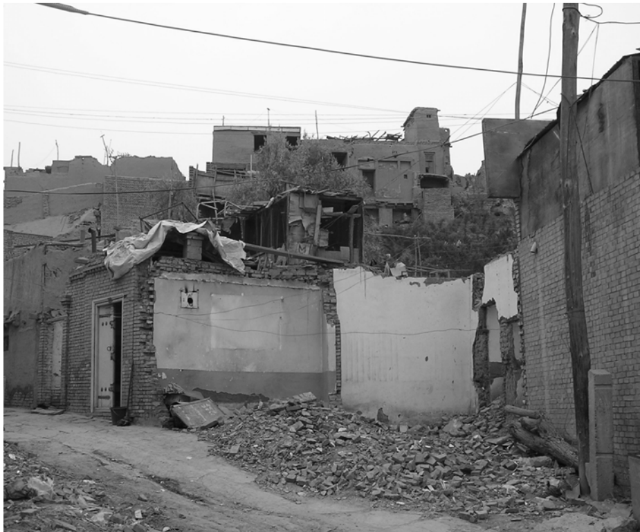
Houses in dilapidated state in old Kashgar
