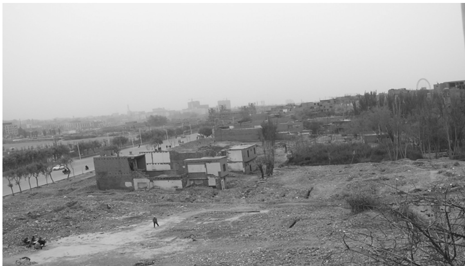
Old houses in old Kashgar town being demolished
